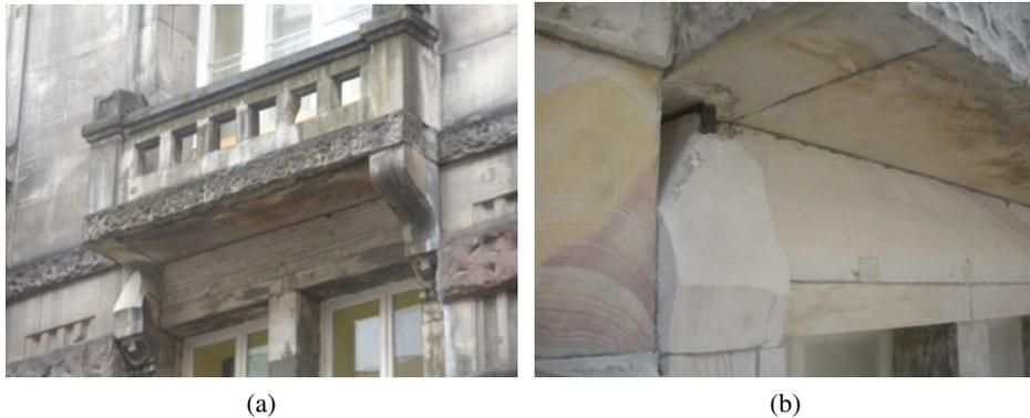
Fig. 11. Warsaw, Kredytowa street 3: a) stone balcony and b) bracket fallen down from the facade
