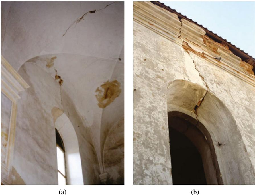
Fig. 9. Synagogue in Słonim, Belarus: a) cracks of the vault and b) the arch above window
