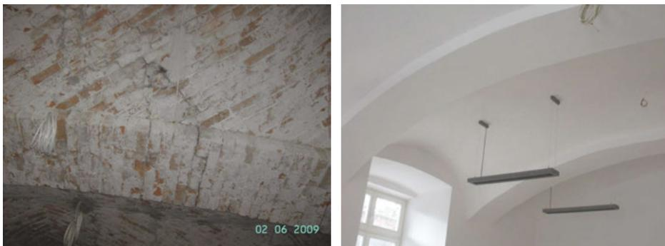
Fig. 6. Royal Palace in Łobzów, Cracow. The vault before (left) and after (right) renovation
