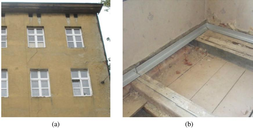
Fig. 8. Tenement house in Łódź, Żeromskiego street: a) cracks on elevation and b) steel bond beam
