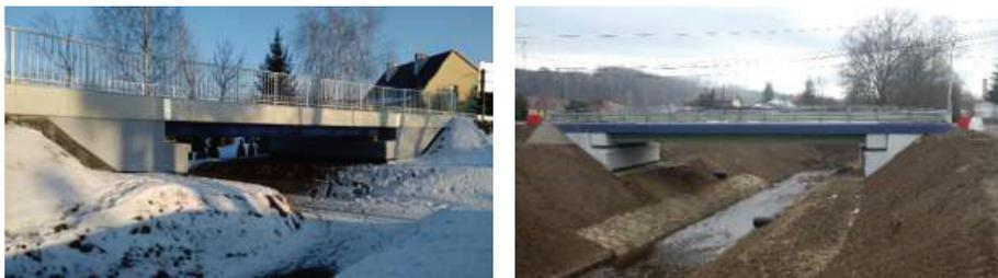
Fig. 8. First Polish vehicle bridges made of FRP materials in service: all-composite (left) and hybrid (right).
