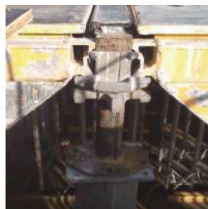
Fig. 4. CC-4 drop head in upper position [10]
