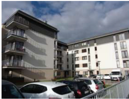
Fig. 1. Multi-family building from 2015. Source: own.
