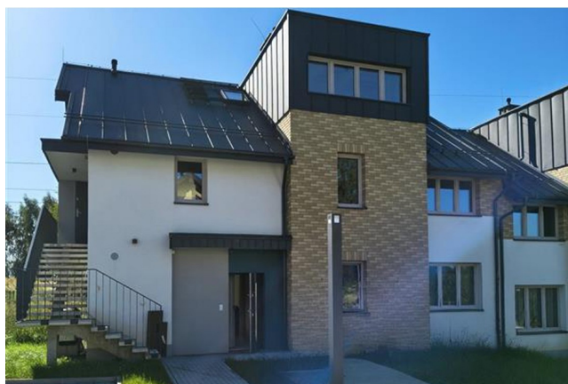
Fig. 1. Front facade of analysed part of the residential building
