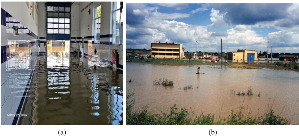
Fig. 6. Causes of bacteriological contamination: a) flooded workshop surfaces (September 2024) – photo by M. Karas; b) a water-filled municipal waste storage basin (July 1997) – archive of the Municipal Services Department in Opole
