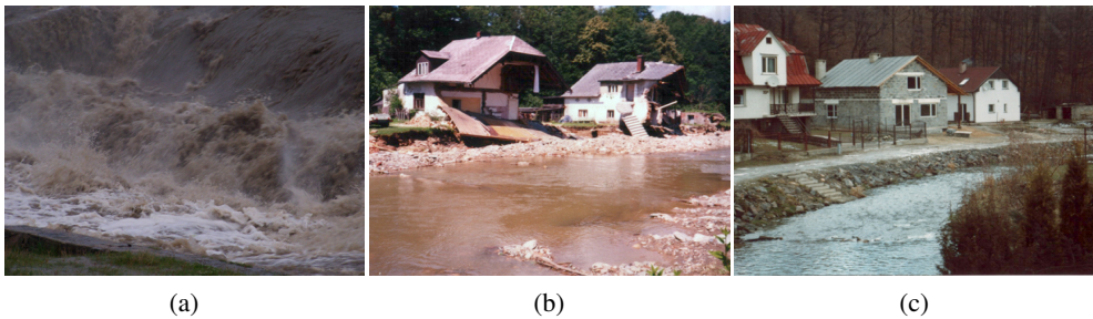
Fig. 2. Residential buildings in the village of Jarnoltówek (near Glucholazy): a) flood wave, b) damaged residential buildings (August 1997), c) newly constructed buildings on the site of the damaged ones (October 1998) – photo by D. Bajno
