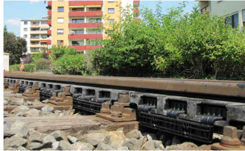
Fig. 23. Application of “dynamic damper” (product of STRAIL Co.)
