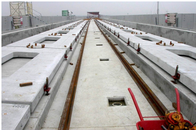
Fig. 8. The ballastless track with prefabricated slab of track in HSR in Taiwan
