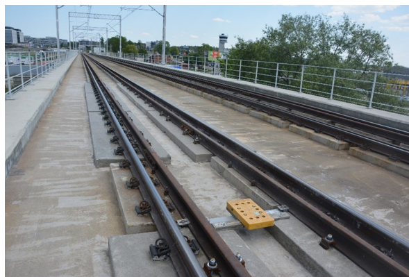
Fig. 2. The ballastless track on the viaduct in Gdańsk, Poland
