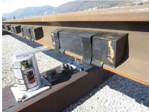
Fig. 22. “Dynamic damper” (product of TATA Steel C)
