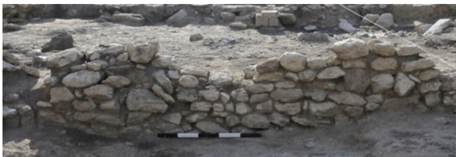
Fig. 3. View of a masonry wall on earth-based mortar, Tanis (Department of Fundamentals of Building WUT archives)
