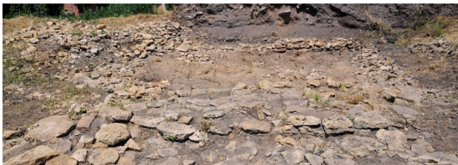
Fig. 2. View of a masonry wall on earth-based mortar, Tanis (Department of Fundamentals of Building WUT archives)
