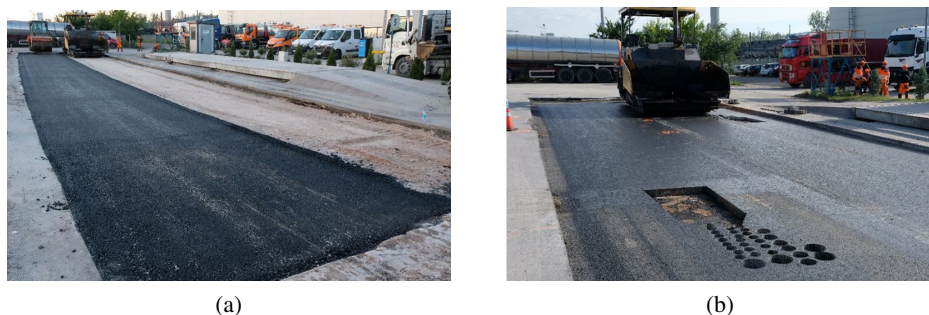
Fig. 6. Construction of the experimental road section: a) Construction of the subbase layer from the HMAC mixture; b) Location of taking samples for testing from the subbase layer
