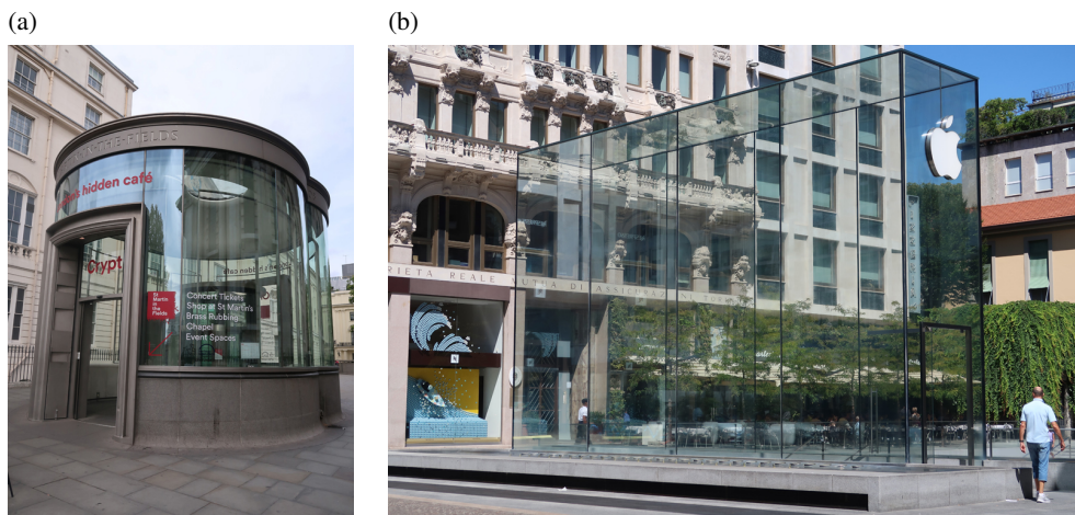
Fig. 1. Load-bearing glass walls in pavilions: (a) Crypt entrance of St Martin-in-the-Fields in London, (b) Apple retail store entrance in Milan (photo by A. Jóźwik)
