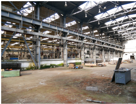
Fig. 7. The junction between the old and new production hall, different types of construction are visible, photo: M. Czarnecki, 2021
