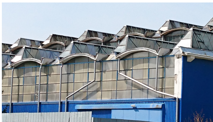
Fig. 1. View of the hall of the Warsaw Pump Factory, photo: M. Czarnecki, 2017
