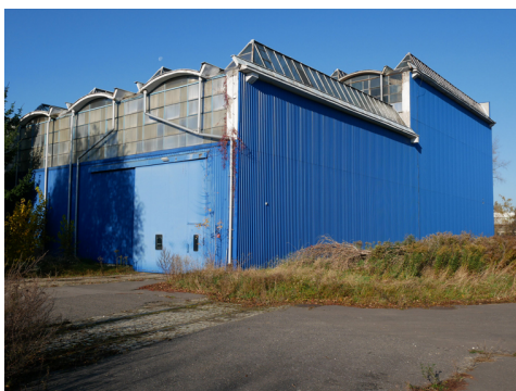
Fig. 2. Production hall building – view from outside, photo: M. Czarnecki, 2021
