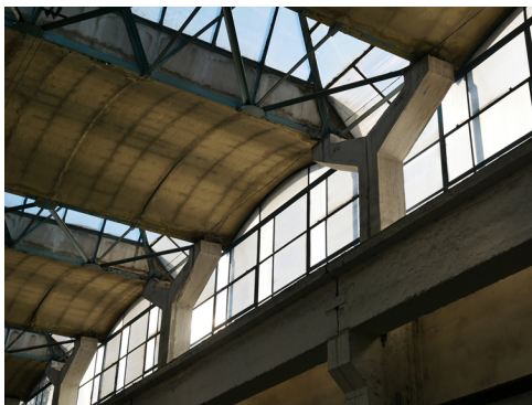
Fig. 5. Reinforced concrete columns carrying steel trusses which provide the support structure for prefabricated thin-walled shell panels, photo: M. Czarnecki, 2021
