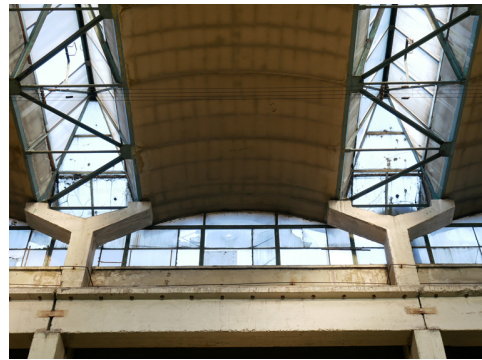
Fig. 8. Detail of the system of hall structures and illumination, photo: M. Czarnecki, 2021
