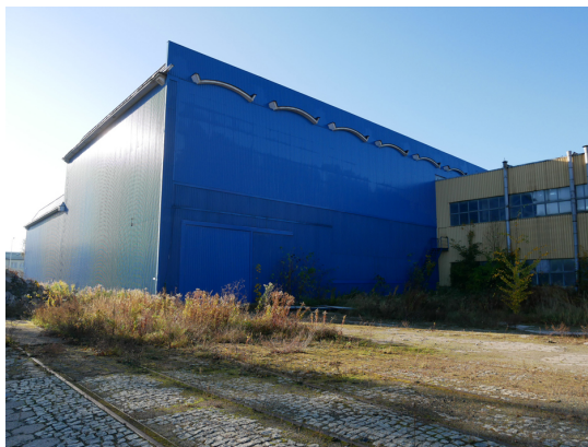
Fig. 4. The original hall covered with sheet metal cladding, on the right the adjacent new hall building, photo: M. Czarnecki, 2021
