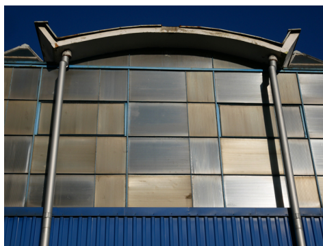
Fig. 3. Detail of glass façade and roof structure from outside, photo: M. Czarnecki, 2021
