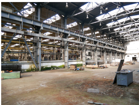
Fig. 7. The junction between the old and new production hall, different types of construction are visible, photo: M. Czarnecki, 2021
