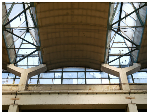
Fig. 8. Detail of the system of hall structures and illumination, photo: M. Czarnecki, 2021
