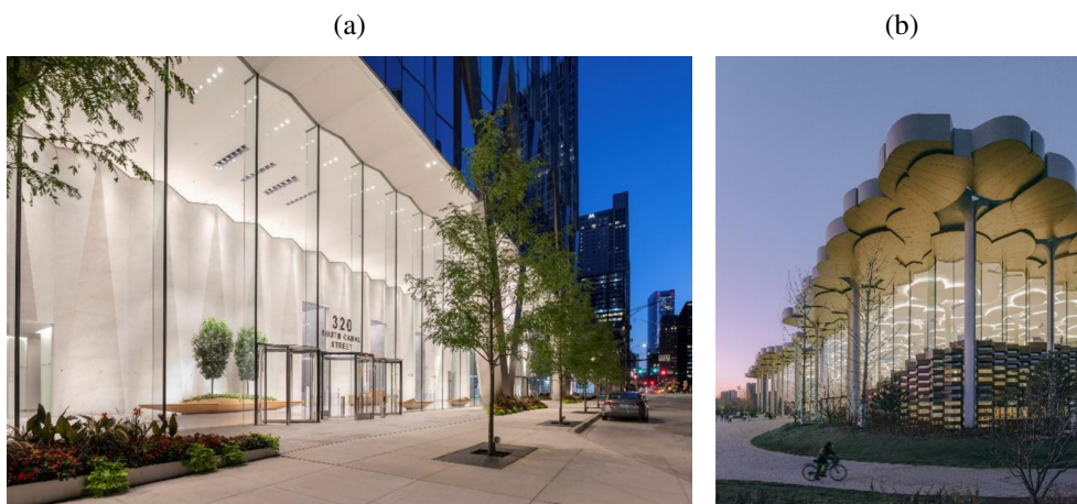
Fig. 8. All-glass facades: (a) glass fins in skyscrapers 320 South Canal in Chicago, architectural project by Goettsch Partners (©Nick Olivieri Photography), (b) glass panels in Sub-Center Library in Beijing, architectural project by Snøhetta (©Zhu Yumeng)
