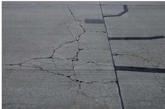
Fig. 1. Damaged LWS concrete slab qualified for replacement [1]
