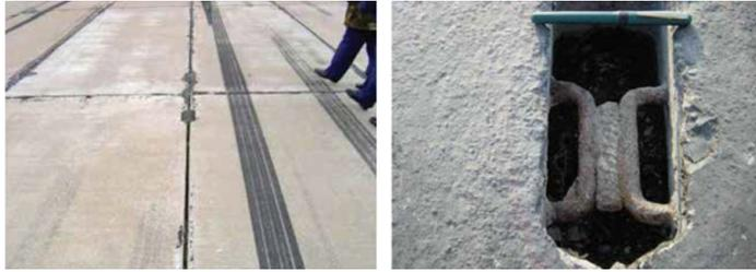
Fig. 4. Connection of LWS slabs using anchors (5 mm expansion joints visible in the left photo) [2]
