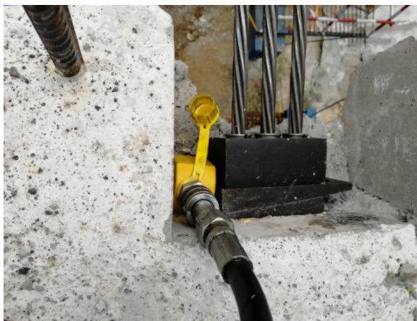
Fig. 8. Special oil pressure jack jacking device
