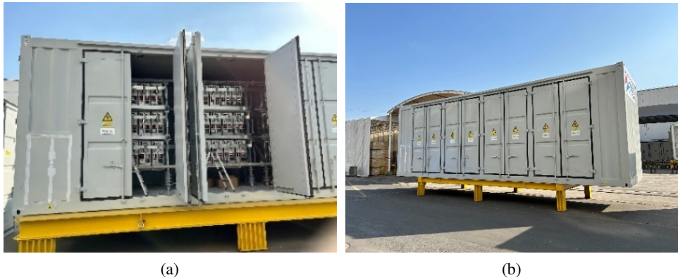
Fig. 1. (a) Space-occupying equipment installed in modular cabin; (b) Equipment-modular integration with large flexible wall-openings
