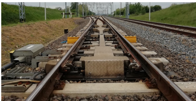
Fig. 8. Turnout 60E1-1200-1:18,5 in single-point machine system with coupling
