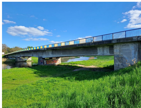
Fig. 1. View of the bridge [own archive]
