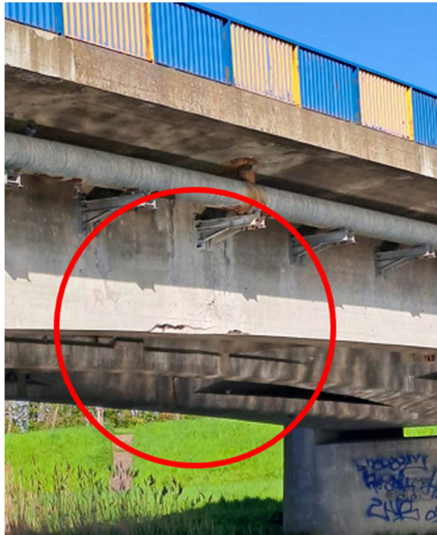
Fig. 12. View of girder 1 in the strand bay. Concrete defects and numerous cracks in the bottom zone of the girder
