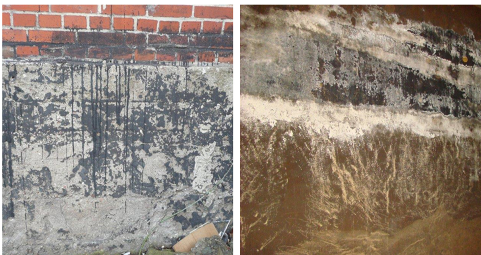
Fig. 4. Reinforced concrete wall of tank from outside and inside with leaks of white efflorescence
