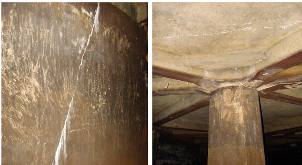
Fig. 5. Wall and pillar supporting rib-and-slab floor. Visible cracks filled with white compounds
