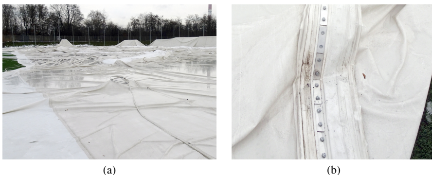
Fig. 5. Condition of the membrane after the disaster – December 23, 2022: (a) coating lying on the turf, (b) tearing of the plating outside the connection
