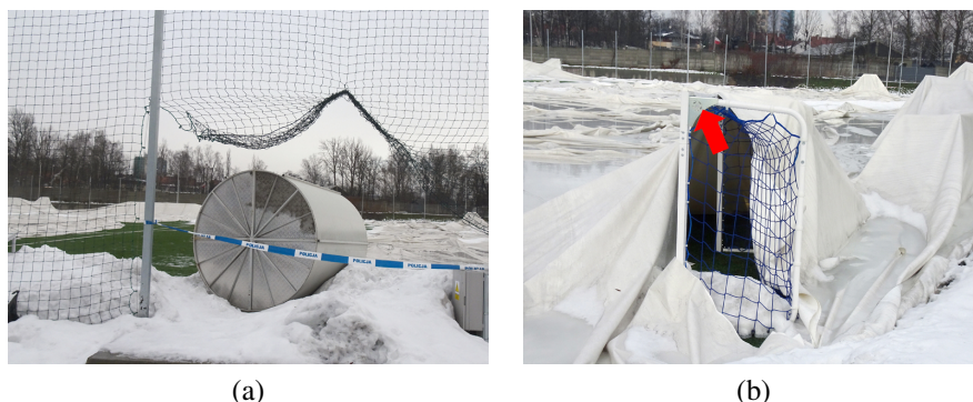
Fig. 6. View of the facility after the disaster: (a) overturned entrance revolving door, (b) tearing of the covering on the edge of the sports goal
