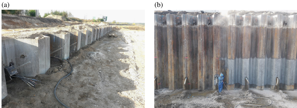
Fig. 2. View of the retaining wall: (a) visible anchor heads; (b) during construction works, front view
