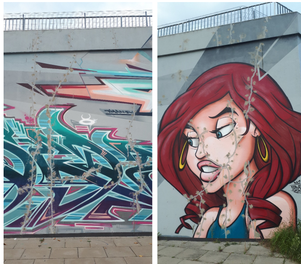
Fig. 4. Traces of repairing the retaining wall (ca. 5–6 m high) defects (vertical cracks); the wall is located along the reservoir's eastern part (photo by T. Godlewski)
