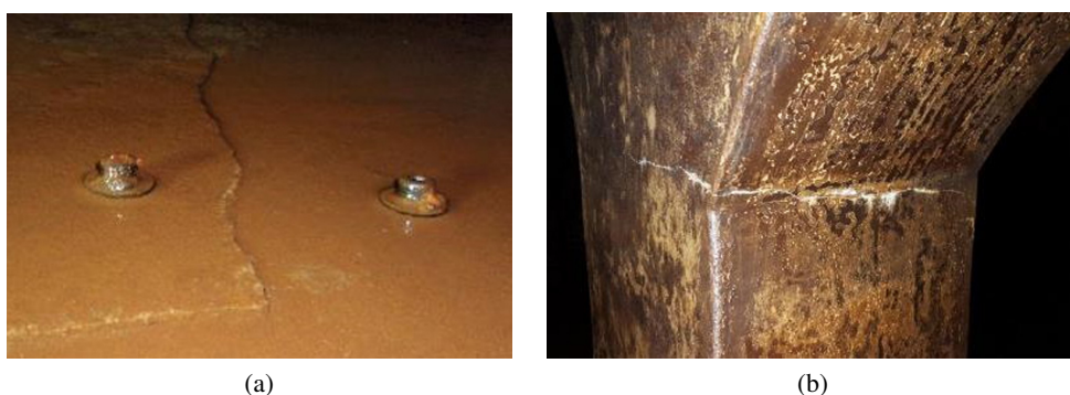
Fig. 7. (a) Bottom plate in the G-F/9-10 axis in chamber I – monitored gap in the repair area, opening width > 2 mm, vertical displacement (offset) visible; (b) column in the H/2 axis (view from axis 3 side) in chamber I – a horizontal tight crack at the column widening area, reaching no further than half the column width (< 25 cm), crack opening ca. 4 mm wide with efflorescence (photo by T. Godlewski)
