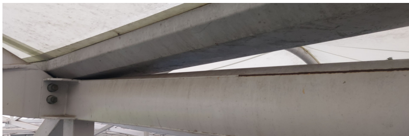
Fig. 4. Deformation of the tubular profile of the second damaged girder
