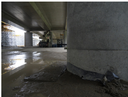
Fig. 7. Deformation and local depression of the working platform near one of the supports
