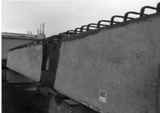
Fig. 4. Two-dimensional code display of prefabricated components
