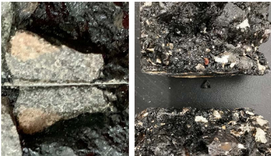
Fig. 6. Physical image of fatigue cracking: (a) Symmetric fatigue cracking of asphalt mixture, (b) Fatigue cracking cross section
