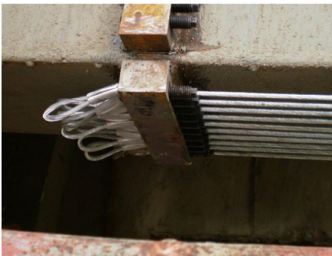
Fig. 11. Wire rope anchorage
