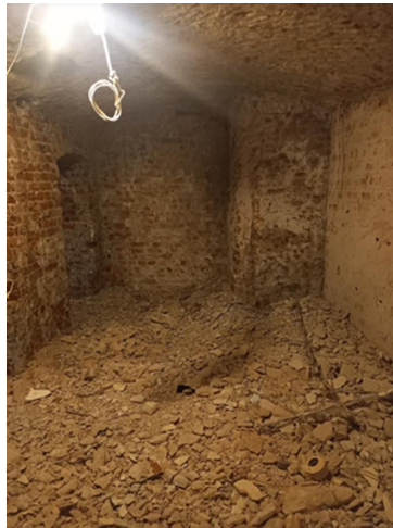
Fig. 1. Demolition works related to the chipping off of plasters
