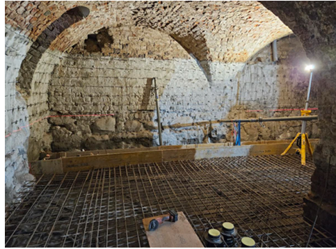
Fig. 2. Construction of a reinforced concrete floor slab and waterproof insulation of walls
