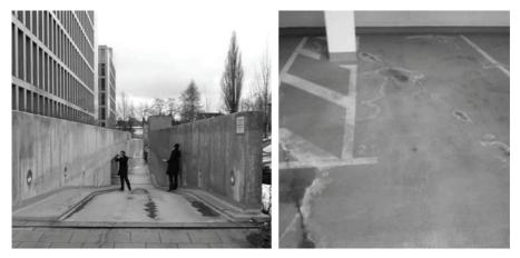
Fig. 5.1.1: APPLIANCE, Bottom Slab in an Underground Parking Lot Loss of tightness due to wide through cracksa) Entrance ramp, b) Wide through cracks with leaking ground water
