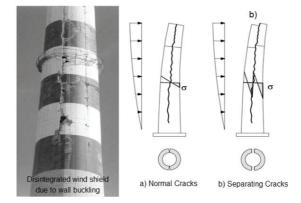
Fig. 1.1: BACKGROUND, Threats by wide separating cracksLoss of the wind load bearing capacity due to wide separating cracksa) Normal cracks due to enough hoop reinforcement, Regular vertical stressesb) Separating cracks due to insufficient hoop reinforcement, Increased vertical stresses
