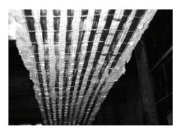
Fig. 5. Ruredil X Mesh Gold after fitting
