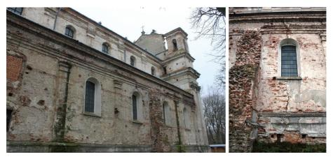
Fig. 7. The photograph depicts the building from the eastern side (photograph to the left). Visible damage of the abutment of the wall, along with the material and structural degradation of the wall (photograph to the right).
