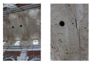
Fig. 5. A view of the cracks and marks on the vault ceiling (photograph to the left), as well as a close-up of the damage (photograph to the right)
