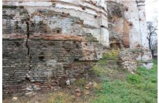
Fig. 10. View of the vault of the main nave walls after the failure associated with the collapse of the structure of the roof due to a fire that occurred in the past.
