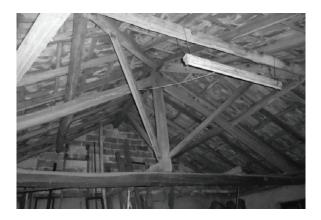
Fig. 16. Covering Structurally Supported by Wood Trusses
