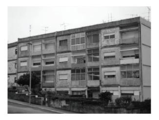
Fig. 5. Portuguese Building Needing Exterior Walls and Window Frames Rehabilitation
