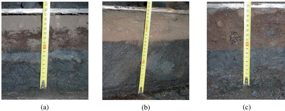
Fig. 2. Tank base with damaged foam glass, 80–160 mm thick
