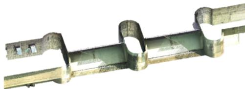
Fig. 2. Results of Besko Dam measurements, model of the external surfaces of the dam [19]
