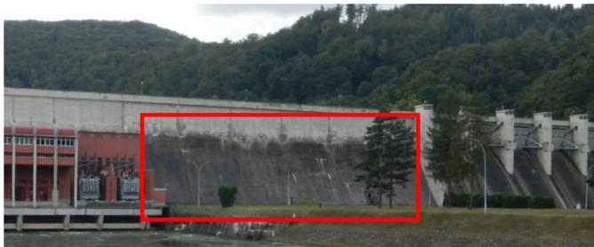
Fig. 10. View of the tested downstream wall of the Rożnów dam with the measured fragment of the wall marked with a red rectangle
