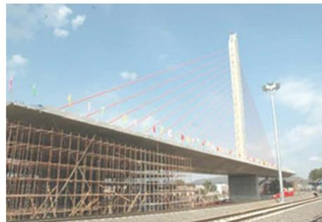
Fig. 2. Support dismantling and swivel of the beam
