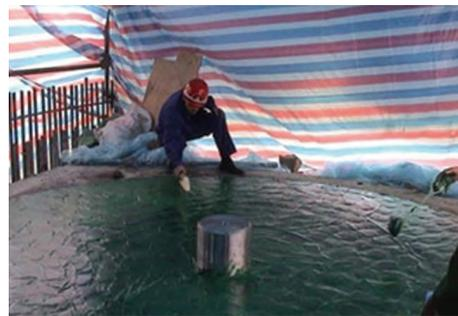
Fig. 1. Location and installation of vinyl plate
