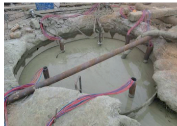
Fig. 2. Pile foundation concrete pouring completed
