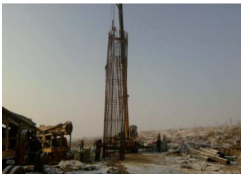
Fig. 1. Lifting reinforcing cage
